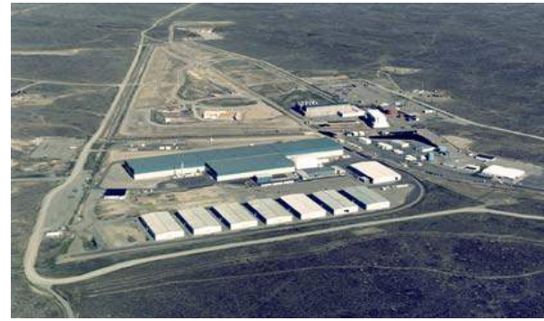
Nuclear Waste Management Complex, Idaho
